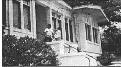
Top: Chapel building. Above: Girls' dormitory converted into educational and office building.
